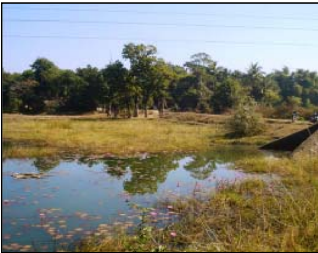
Silted part of Dantiamunhan canal
