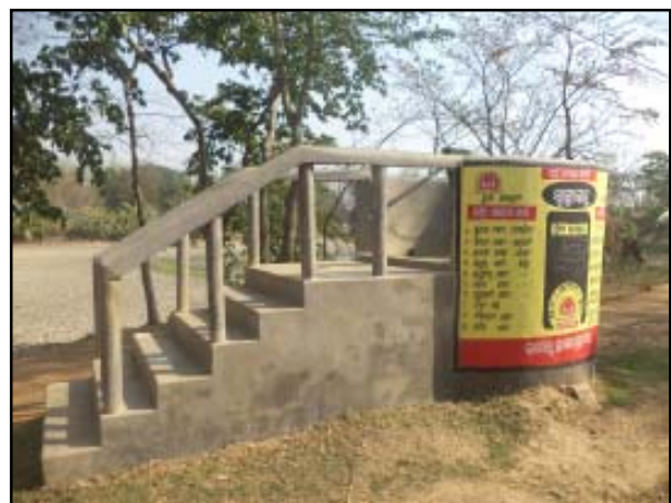
Raised Tube Well with the support of Oxfam
